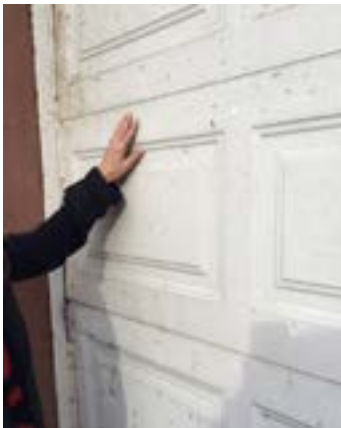
Current retractable door with vinyl surface
