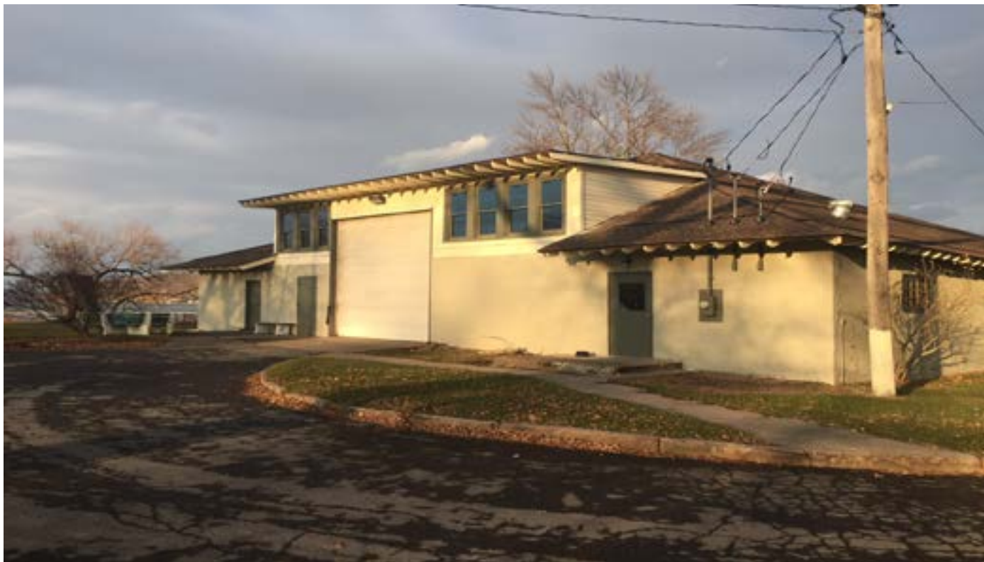
New roof and new west facade windows on Wharton Studio building -- fall 2017
